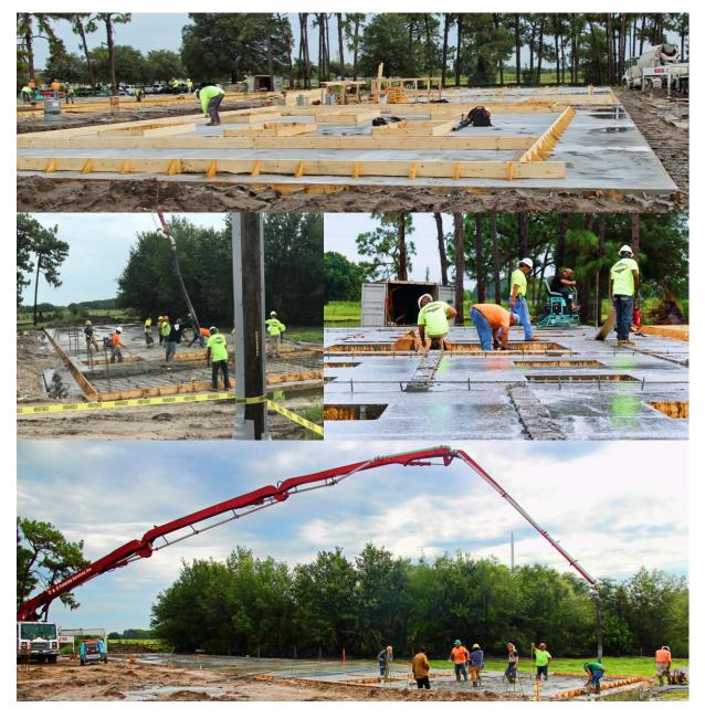
The construction of the new Residence Hall is underway full-speed. The walls are being formed on the ground (see above) to be lifted into place by cranes on August 21 (see press release below). This three-story facility will house 90 students and house parents. All resident students will be on campus when it is completed, bringing our college community closer together. There will be common areas for students to socialize and work on projects together.
